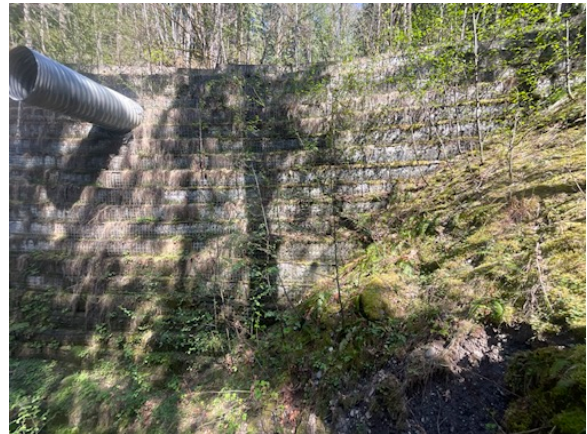
High wall with no signs of deformation.
