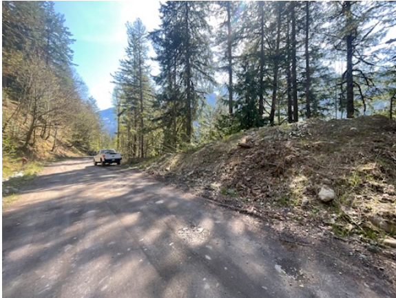
Town approach, remove spoil pile
